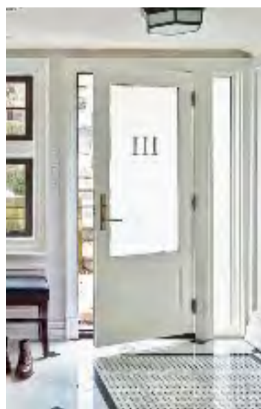
The Summerhill home entrance retiled and pointed post-renovation.
